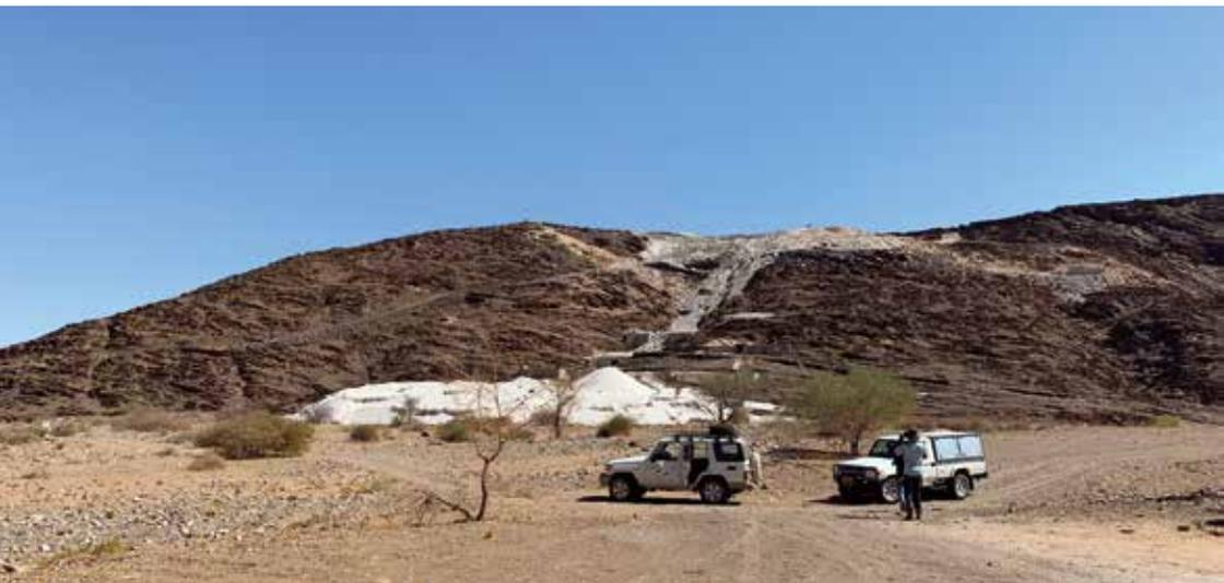
*Figure 21: Tailings of historic mining activity at De Rust pegmatite (Photo: BGR-GSN-Project 2019).*
