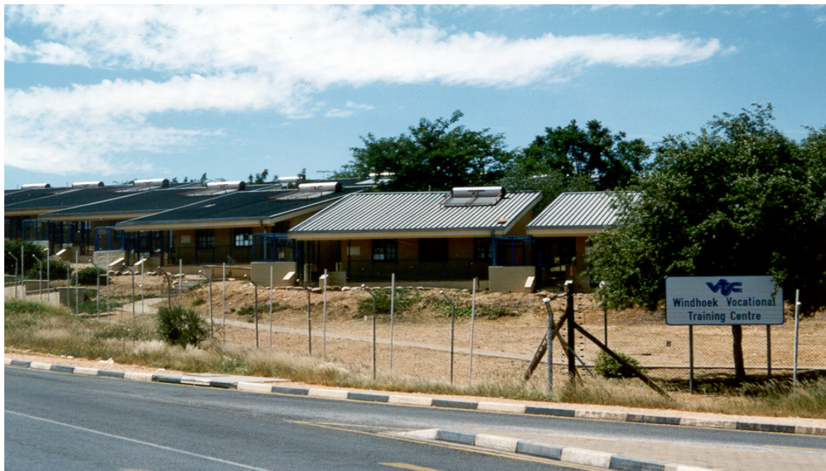
Solar Water Heaters
