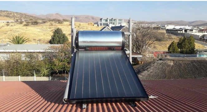
A Solar Water Heater uses energy from the sun to heat water for domestic use.
