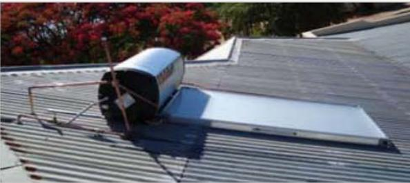
A **Solar Water Heater** uses energy from the sun to heat water for domestic use.
