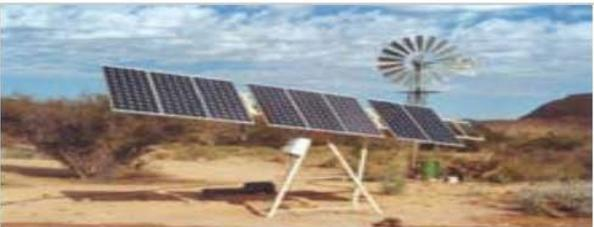
A **Solar Water Pump** uses solar photo-voltaic panels to provide energy for pumping water for livestock and domestic use.
